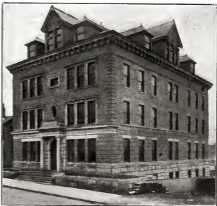
INDUSTRIAL SCHOOL, HOMESTEAD, PENNSYLVANIA Built by Mr. Schwab
